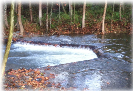
Portage Creek crossvane, located upstream of the mouth of Salt Run
